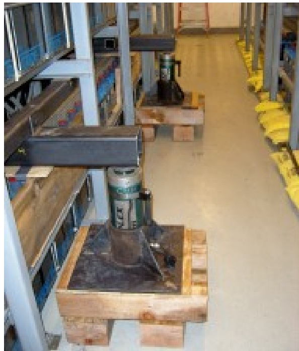
Single rack rams in place
