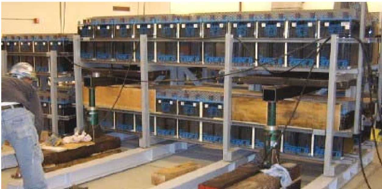
Lift complete – W6 steel installed
